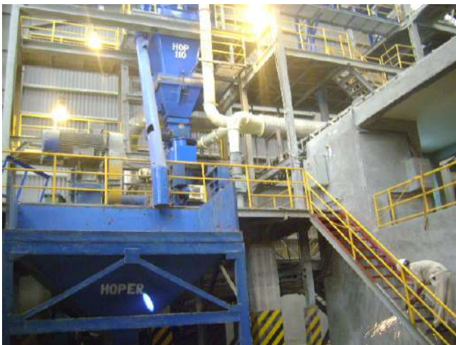
Figure 1. View of the compactor E72.
